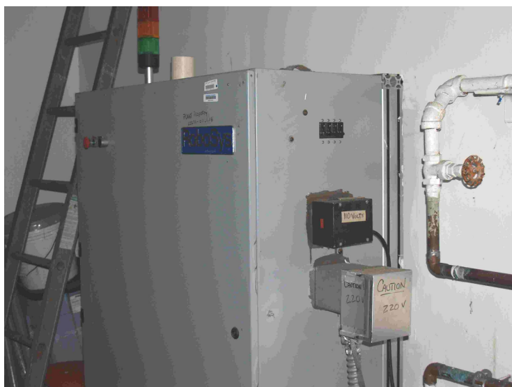
Figure 45 Filter Installation to Suppress Motor-Controller Noise
