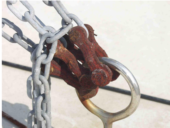
Figure 16 Example of a Rusty Joint
